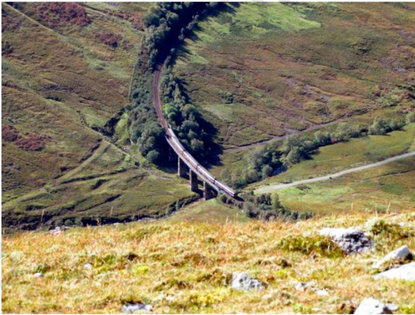
Fig 4. Glen Coralan Viaduct/West Highland Line. Photo Brian Davey
